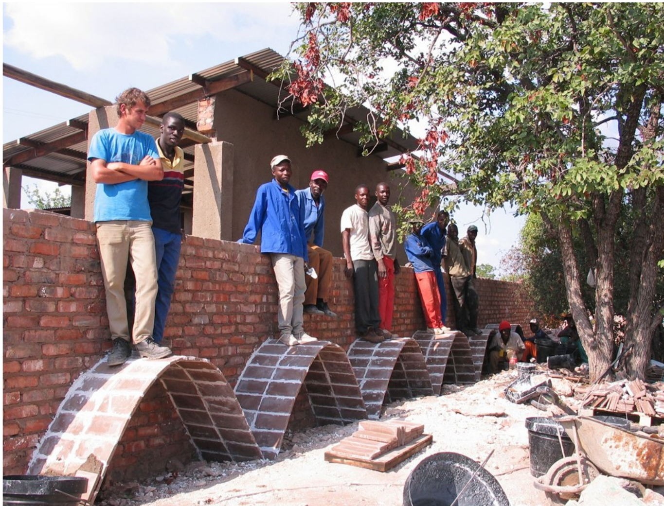
Figure 7 - workers test vaults
