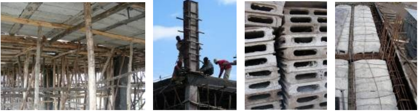
Fig. 8. A selection of imported – hence expensive – building materials in current “low-cost” projects: a) Precision timber for formwork; b) precision formwork for columns and edge beams; c) interior panels (Made in China); and d) reinforcement steel and Portland cement for concrete.
