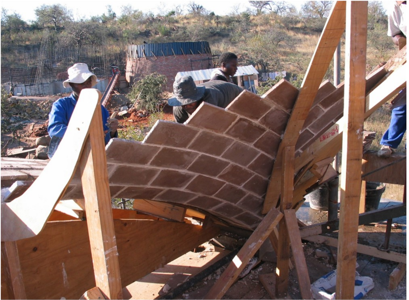
Figure 6 - Headquarters under construction
