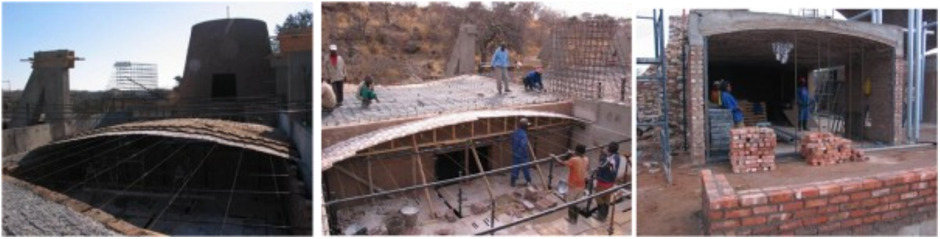
Fig. 8. The floor system in the Mapungubwe project uses a) structural vaults as permanent formwork for b) a mass concrete floor. c) This floor can be built without formwork and significantly reduces the amount of reinforcement steel necessary. In the Mapungubwe project, the edge beams are made in reinforced concrete. (Image credits: James Bellamy.)
