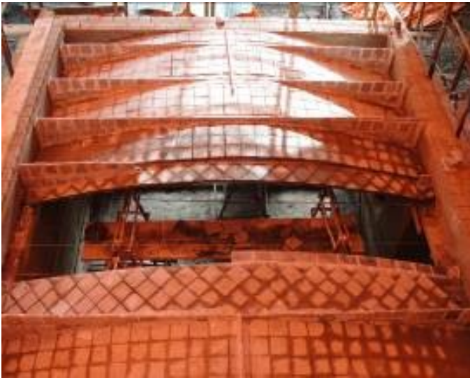
Fig. 6. Unreinforced thin-tiled floor system of housing prototype for Ethiopia: simple, single-curved barrel vault with stiffeners (Image credits: Lara Davis).
