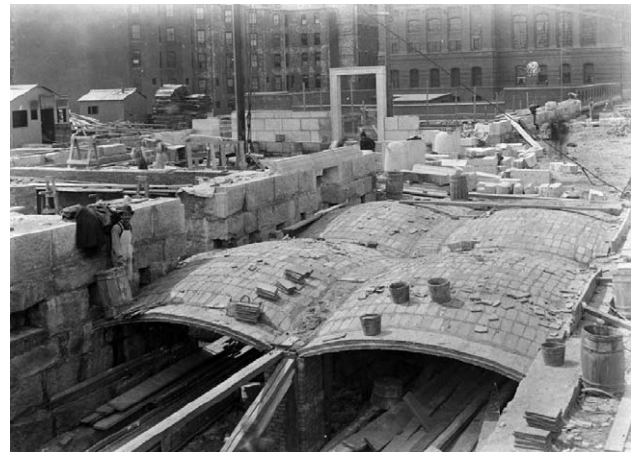
Fig. 3. a) Rafael Guastavino standing on a newly built arch during construction of the Boston Public Library, Boston, Massachusetts, 1889. [10] b) Guastavino Rib and Dome System, New York, 1902. [11]
