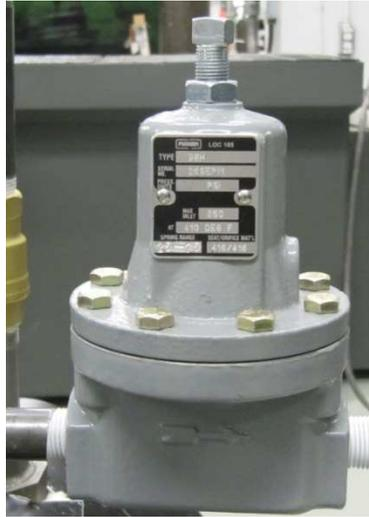
Figure 40: Back Pressure Regulating Valve
