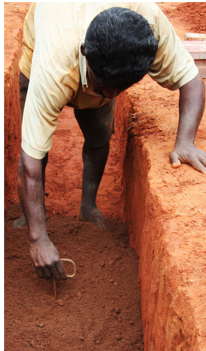
Checking the layer thickness
