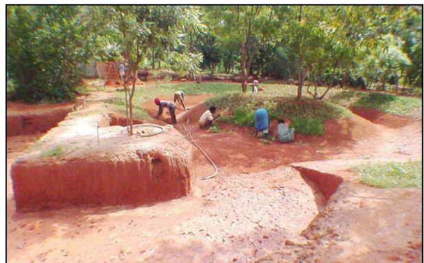
Laying back the top soil and planting grass
