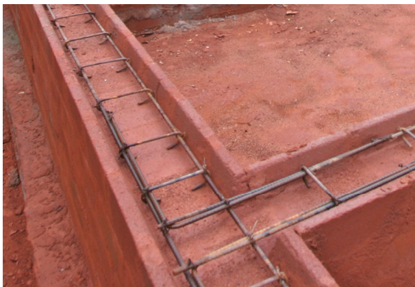
U blocks 240 of the composite plinth beam
