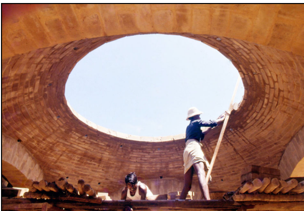
Building hemispherical dome on pendentives
