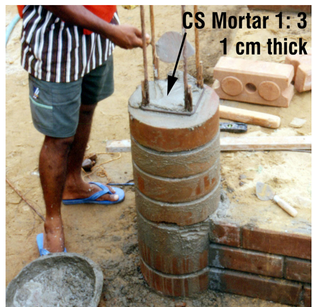
Laying mortar and stirrups
