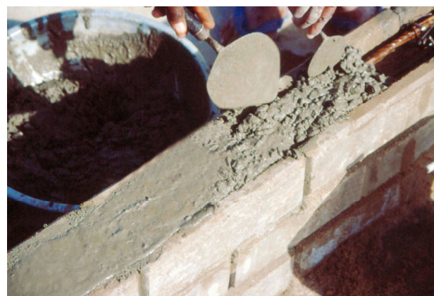
Casting concrete in the composite plinth beam 290
