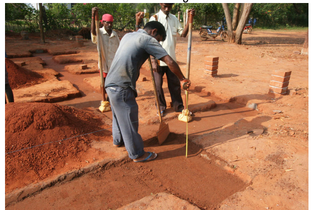
Checking the level of the foundation
