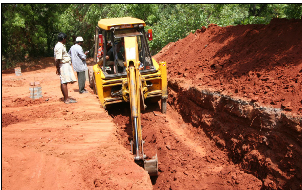
Excavation with an excavator first
