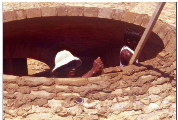
Checking blocks with a compass
