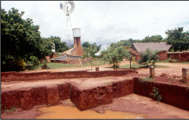
Excavation of the basement, 1.2 m below ground level
