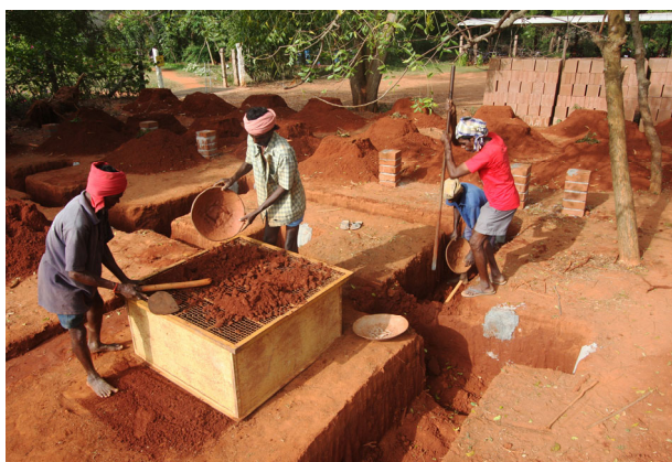
Digging the trench foundations
