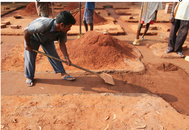
Scraping the top to level the foundation
