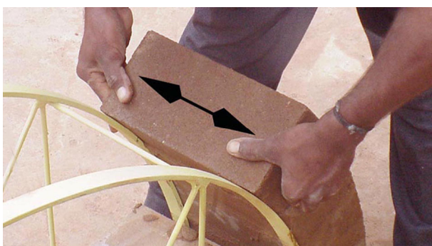
After laying the mortar, slide the block laterally
