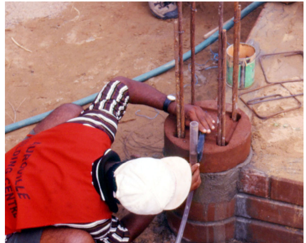
Checking the levels
