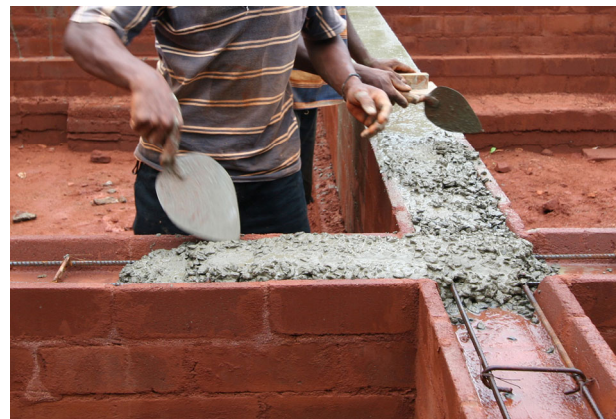
Casting concrete in the composite plinth beam 240
