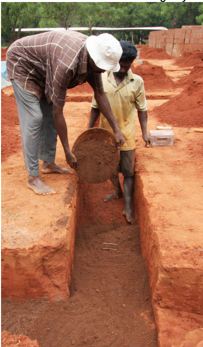
Pouring the mix in the trench
