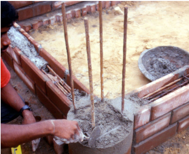
Casting the plinth beam
