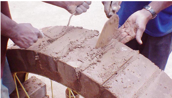
Closing the arch with a very tight mortar
