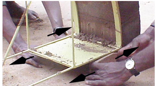
Sliding out wedges progressively for decentring
