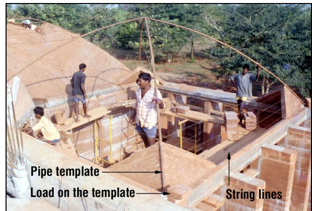
Pipe template and string lines
