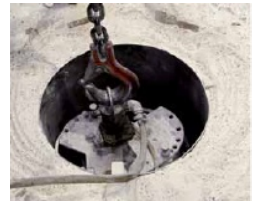
Former vibration tooling
