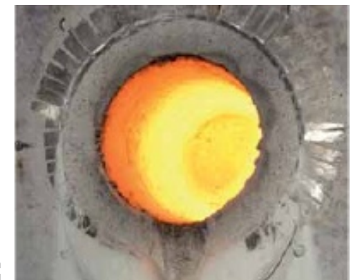
Sintered lining with KELLUNDITE material
