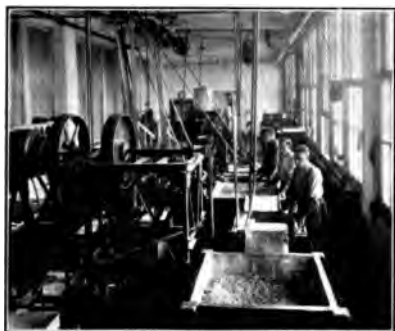
Washing the flake. Centrifugal dryers shown in the background.
