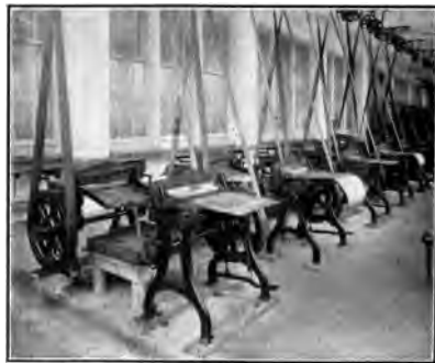
Cutting copper-nickel sheets into 1-16 inch squares. Each square makes 125 nickel "flakes" when the copper is chemically removed.
