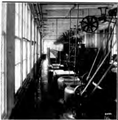
Dissolving copper from small copper-nickel squares.
