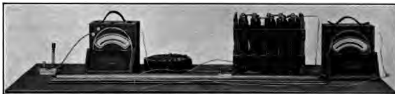
Battery of Small Edison Cells furnishing power for Wheatstone bridge and fall of potential experiments.
