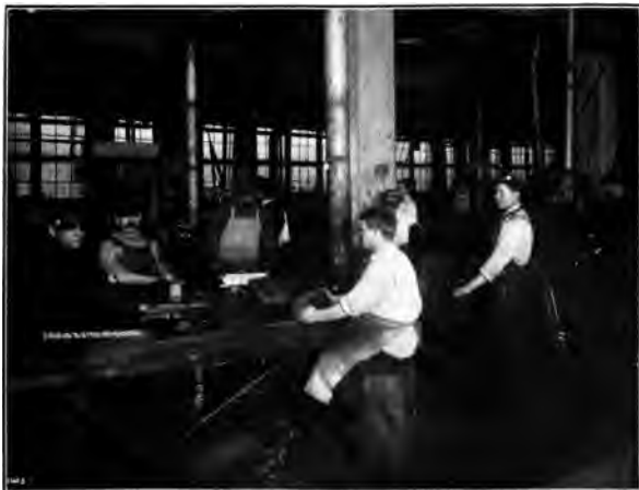
Loading the Negative Pocket with Iron Oxide.
