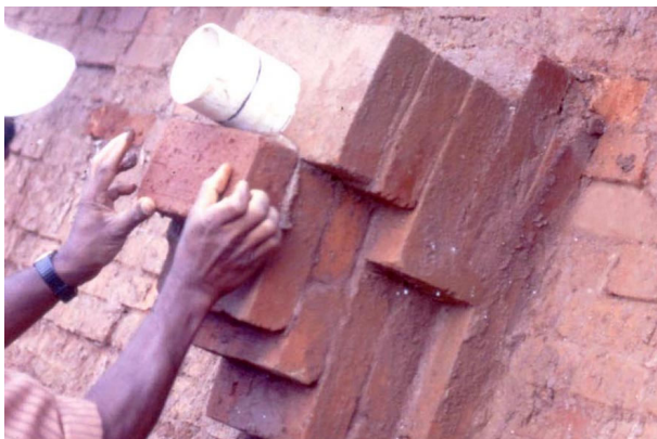
Fig. 166 – Protecting a resonator of 88 cm long
