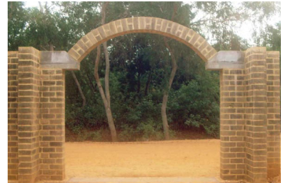
Segmental arch – Auroville
