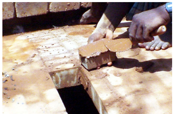
Fig. 138 – Apply 2-3 mm of glue on the block
