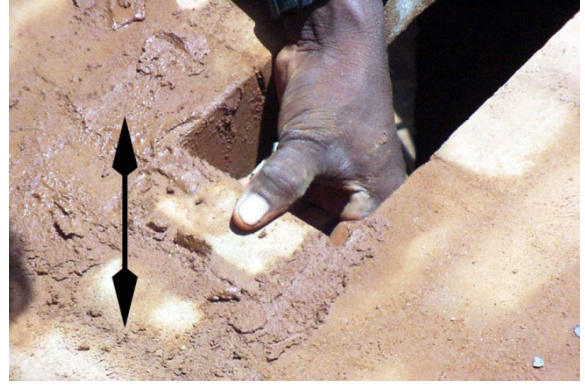
Fig. 140 – Adjust the block by sliding it vertically
