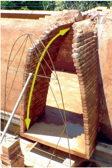
Fig. 110 – Force as a rampant arch
