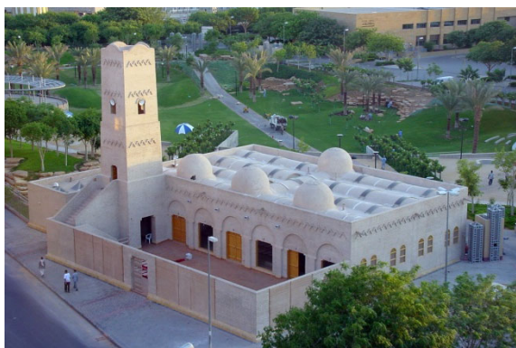
Al Medy Mosque – Riyadh, Saudi Arabia, 2004. Semicircular domes \varnothing 3.01 m, CSEB
