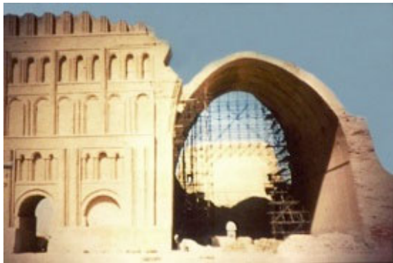
Iwan of the Palace of Ctesiphon – Iraq, ca. 6 th century Vault 21 m span, 30 m high, fired brick
