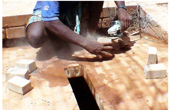
Fig. 137 – Grind a block to adjust its length
