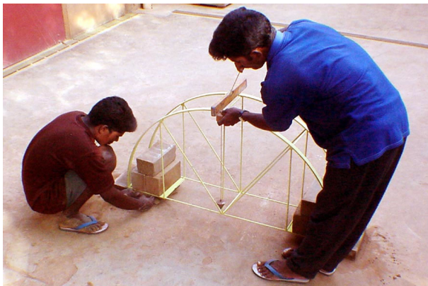
Fig. 125 – Check the level and verticality
