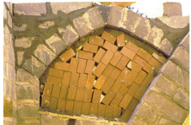
Fig. 123 – Masonry centring, \pm 80 cm span
