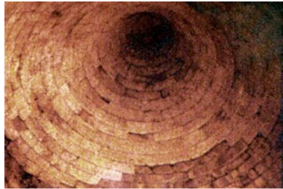
Tomb of Atreus – Mycenae, Greece, 1325 BC Pointed dome ~ Ø18 m, stone
