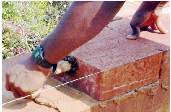
Fig. 150 – Compress the joint
