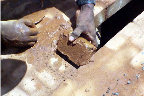
Fig. 139 – Insert the block. Note the mortar on the sides
