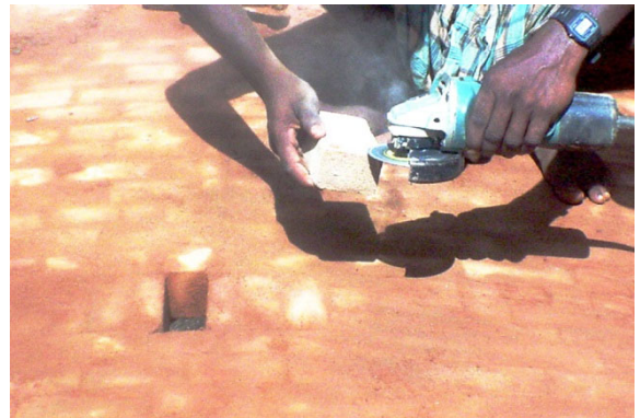
Fig. 142 – Grind the keystone to adjust its thickness
