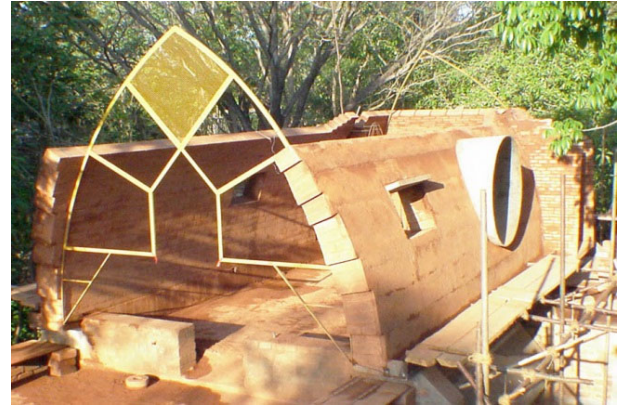
Fig. 116 – Equilateral vault with horizontal courses
