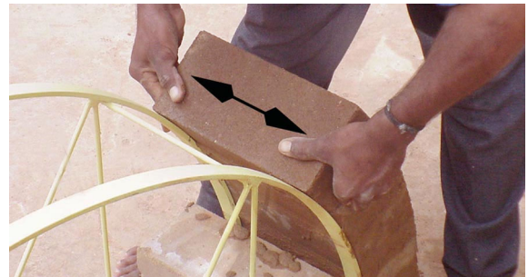
Fig. 129 – Slide the block laterally
