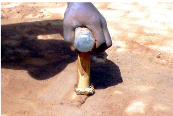
Fig. 146 – Gently hit the keystone to wedge it into place
