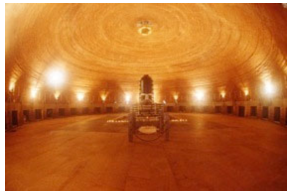
Dhyanalinga Temple – Poondi, India, 1998. Segmental elliptical \varnothing 22.16 m, fired brick
