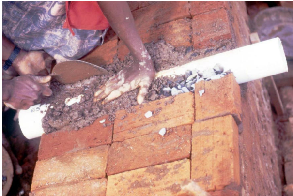
Fig. 164 – Inserting a pipe of 65 cm long
