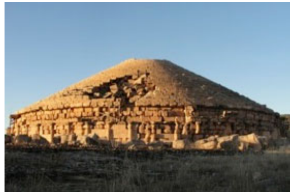
Imedghassen Mausoleum – Algeria, ca. 4 th century BC Corbelled dome ~ Ø58.86 m, stone
