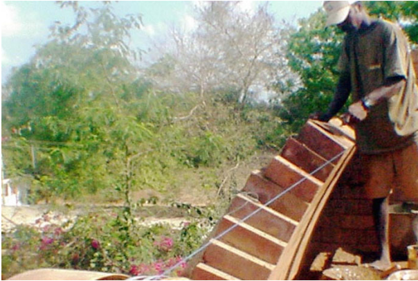
Fig. 106 – The vault rises with horizontal courses
