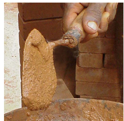
Fig. 120 – 7-8 mm left on the trowel
