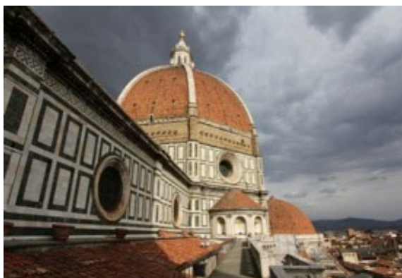
Santa Maria del Fiore – Florence, Italy, 1421-35 AD Facetted dome Ø45.4 m, fired brick
