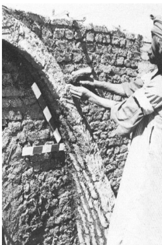
Fig. 105 – Nubian vault construction
