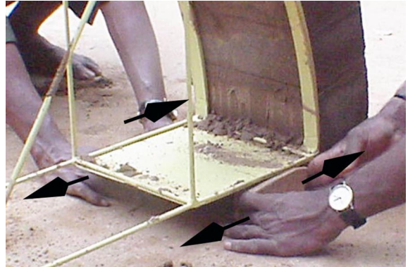
Fig. 131 – Removing wedges and decentring
