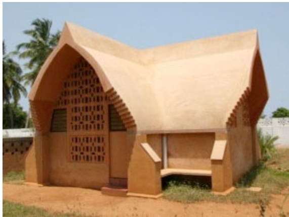
Ermitage – Chinna Kalapet, India, 2006. Equilateral vault 4 m span, CSEB
