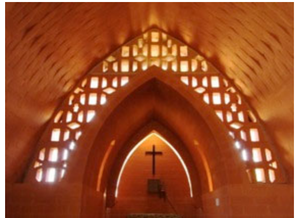
Ermitage – Chinna Kalapet, India, 2006. Equilateral vault 4 m span, CSEB
