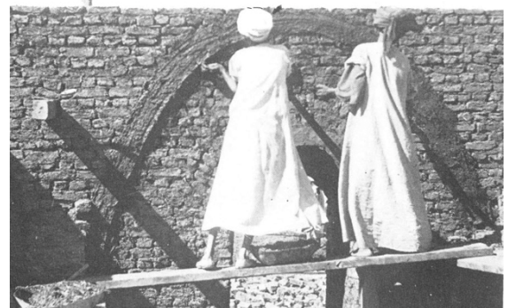
Fig. 104 – Adjusting the curve (Fathy)
