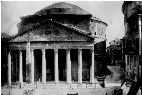
The Pantheon – Rome, Italy, 75-138 AD Dome Ø43.30 m, pozzolan concrete and brick
