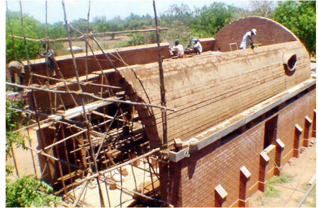
Fig. 107 – Building a semicircular vault of 6 m span
