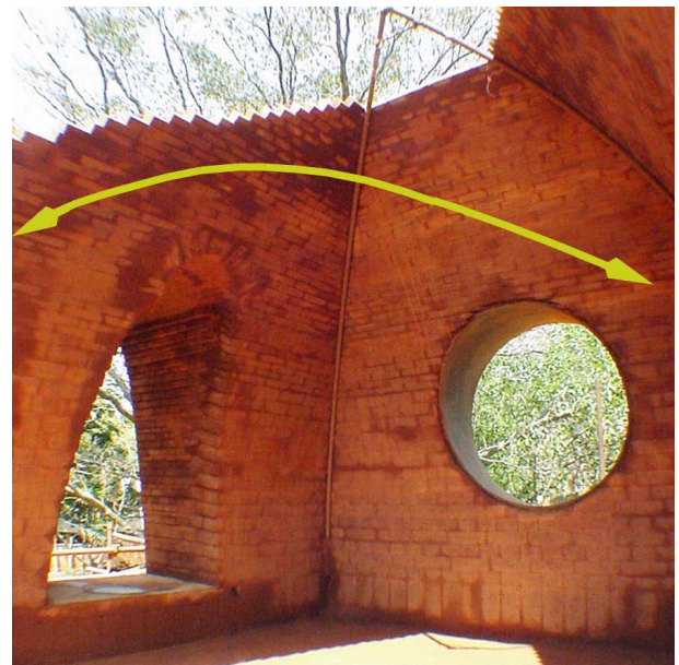
Fig. 109 – Load transfer in the shape of a catenary in an equilateral vault with a half dome
