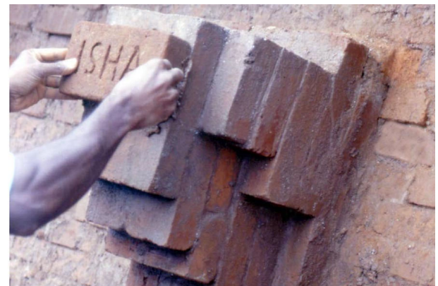
Fig. 167 – Closing a resonator of 88 cm long
