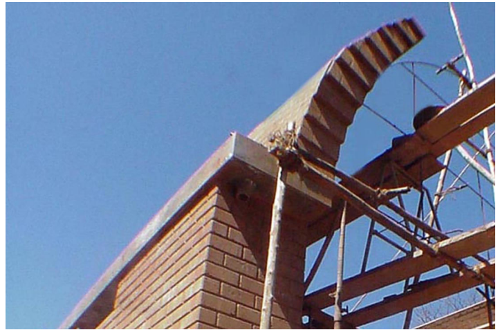
Fig. 113 – Limit of stability of the curved corbel
