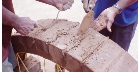
Fig. 133 – Pressing the mortar joint
