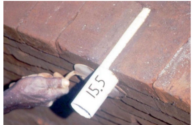
Fig. 165 – Inserting a pipe of 15.5 cm long
