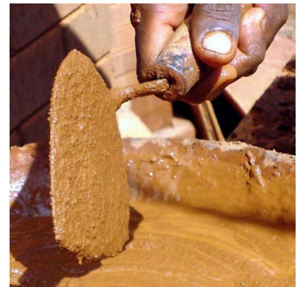
Fig. 119 – 3-4 mm left on the trowel
