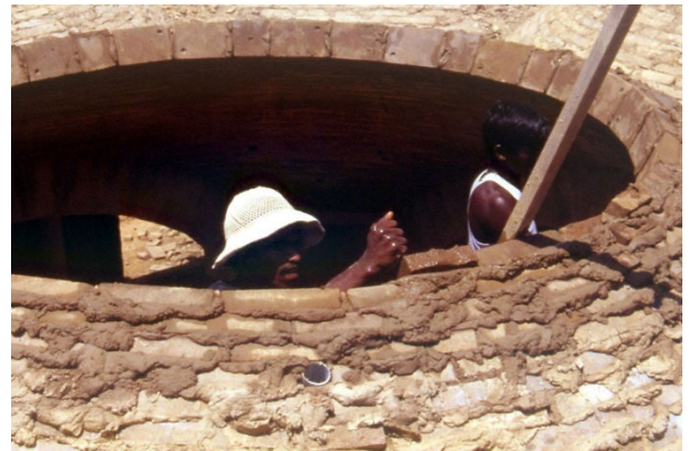
Fig. 153 – Checking blocks with a compass
