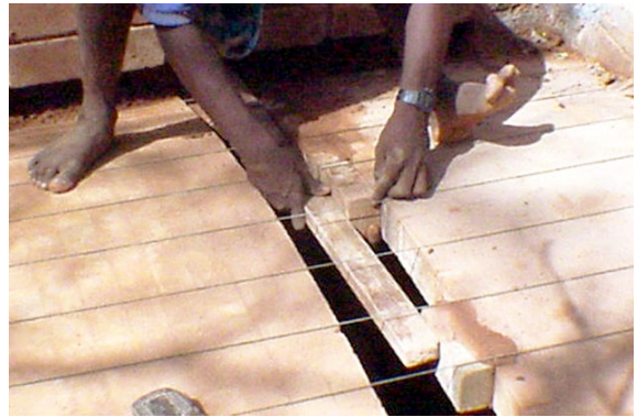
Fig. 136 – Check the linearity of the last course
