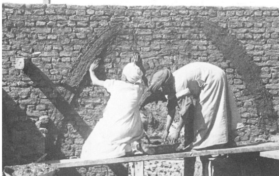
Fig. 103 – Shaping a curve on the adobe wall (Fathy)
