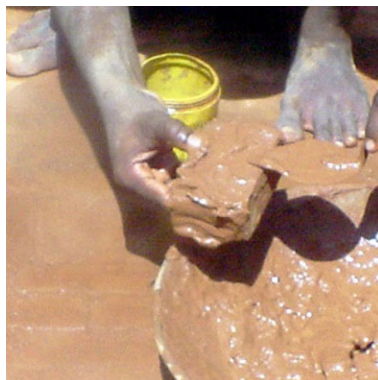
Fig. 144 – Apply 2-3 mm of glue on the 4 laying faces
