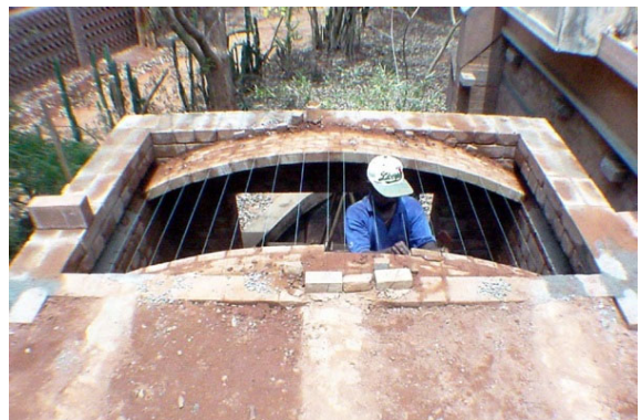
Fig. 135 – Start the vault on both sides
