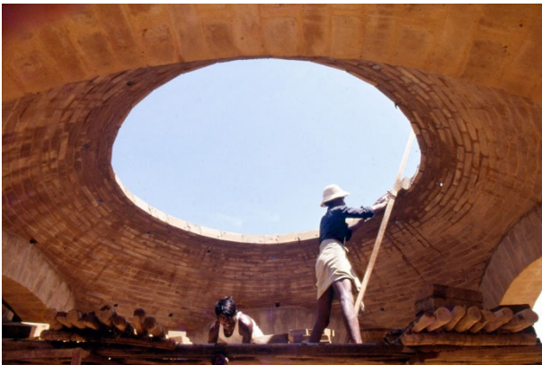
Fig. 152 – Building hemispherical dome on pendentives
