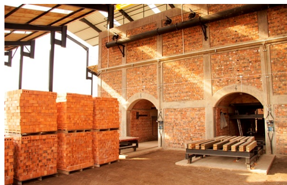
Figure 3: Structure of VSBK by Langkloof Brick, Jeffrey's Bay, Eastern Cape, South Africa.
