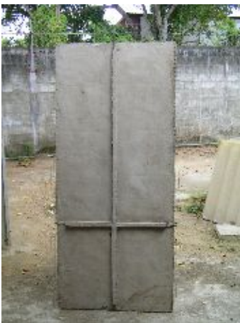
Pre cast panel for five m 3 tanks
