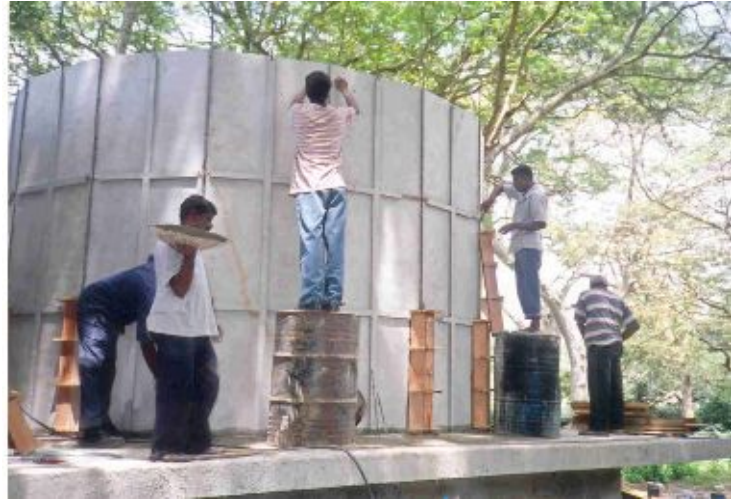
Aassembling work of the 50-m3 tank
