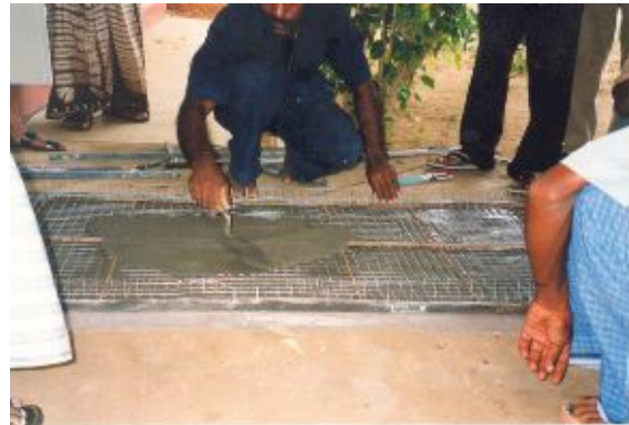
Casting of panels
