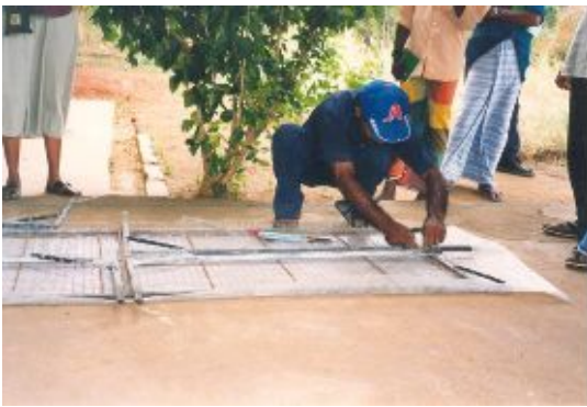
Preparation of mesh and steel for the ribs
