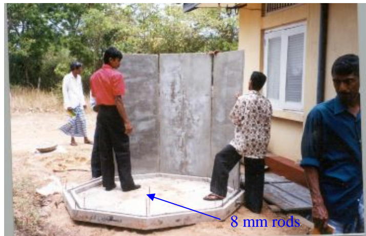
Assembling work on pre cast slab
