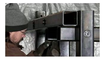
Finally, put the rear upper crossbar on top of the Cant bar and bolt it in place.
