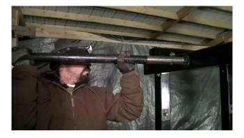
Weld the insert in place. Grind the welds smooth.
