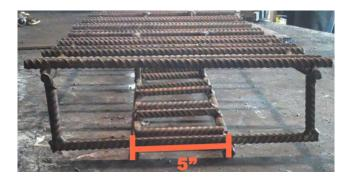
Weld on two pieces of rebar (part WTWJ#6) at either end of the bottom of the welding jig. On top of that, weld two short pieces of rebar (part WTWJ#4) upright. Also, weld six pieces of short rebar (part WTWJ#5) in pairs, equally spaced from one end of the jig to the other. Be sure to weld them outside the pairs of rebar that the track pieces will go inside of.
